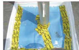
③ Sealing of the support
