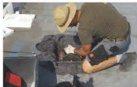
① Opening of the roof cladding
