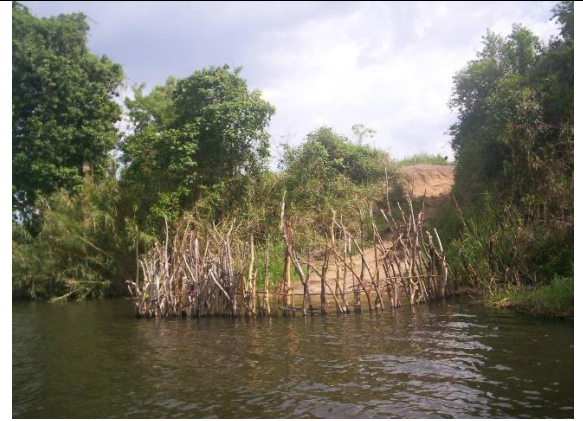
Fig. A.43. Construction of water fetching enclosure to avoid problem C.niloticus habitats, MFNP
