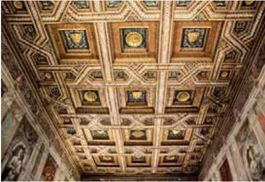
Fig. 34. The coffered ceiling of the Sala dei Cavalli in Palazzo Te, where Charles V was entertained in 1530, with diagonally crossing beams (Foto "Fseveri", in Wikipedia).
