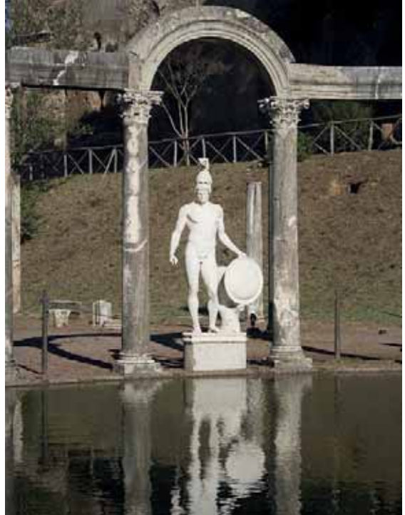
Fig. 30. Detail of the alternating trabeated and arched colonnade surrounding the Canopus of the Villa Adriana, Tivoli (Foto: Gabriele Ferrazzi).
