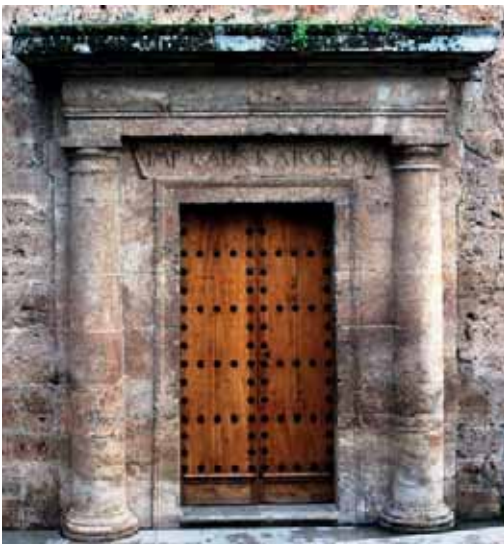
Fig. 31. The northern portal, with Tuscan capitals and bases (now partly hidden) and a Vitruvian portal narrowing towards the top. The pulvinated frieze is effective but unorthodox (Foto Author).
