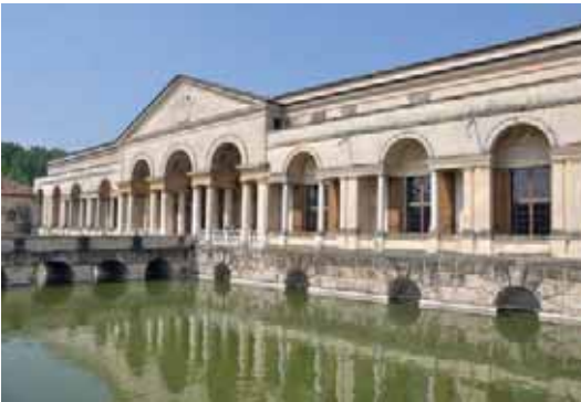
Fig. 36. View of the garden facade of Palazzo Te, Mantua.
