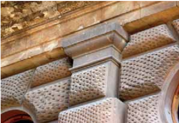
Fig. 20. Detail of the Doric capital and rustication of the Palace (Foto Author).
