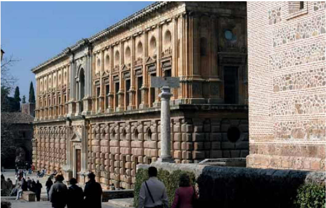
Fig. 3. General view of the south façade of the Palace (Foto Author).
