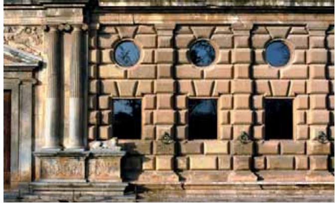
Fig. 19. Detail of the south facade of the Palace (Foto Author).
