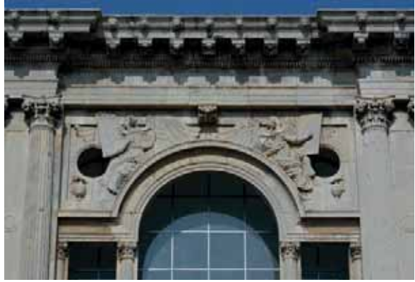
Fig. 27. Detail of the serliana of the southern portal (Foto Author).
