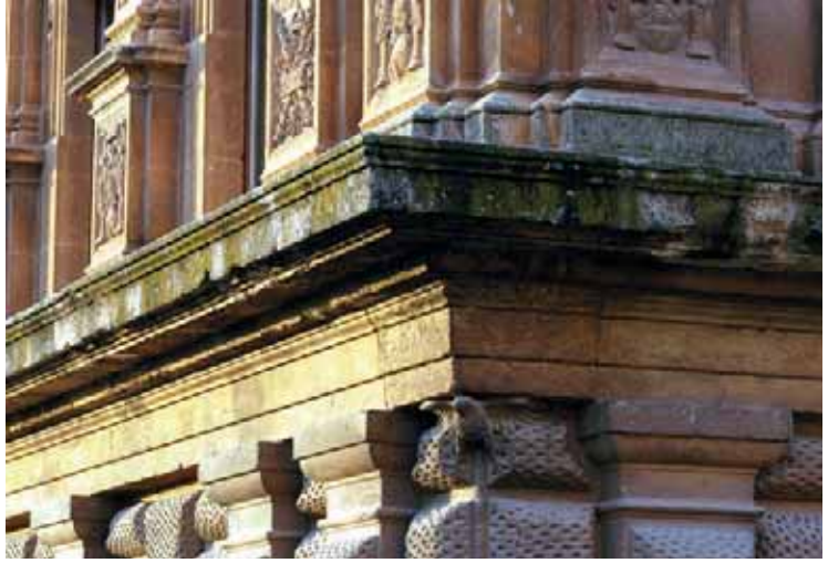
Fig. 9. The southeast corner of the Palace: the pilasters flank the corner (Foto: Author).
