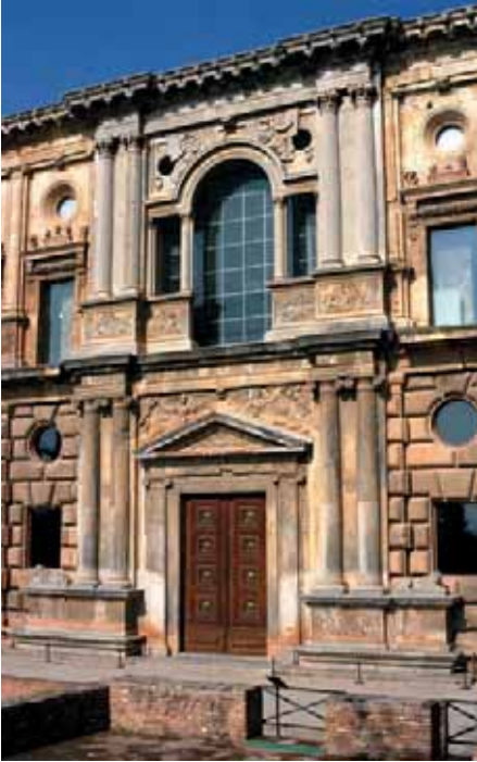
Fig. 26. The southern portal of the Palace (Foto Author).
