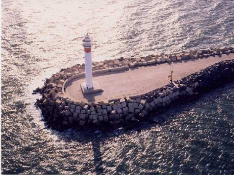
Faro del dique Juan Carlos I. (Foto AAPH)
